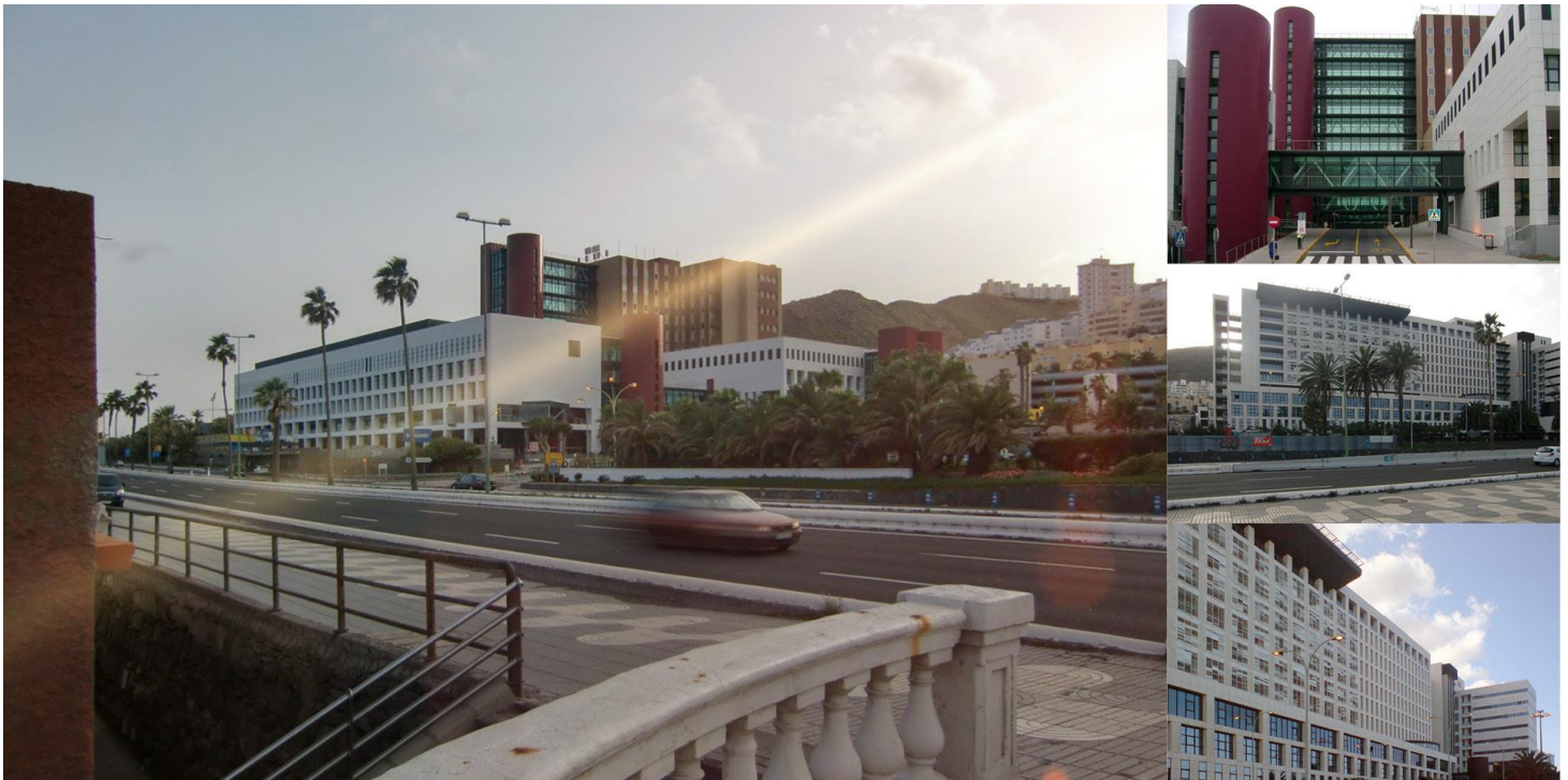
concrete structure, reinforced concrete slabs, columns and walls. steel pedestrian bridge between buildings (872 beds)
